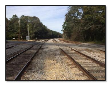
The upgrades include replacing the current worn asphalt crossing with high density concrete panels between the railroad tracks. MSE construction crews will also remove and replace several railroad ties and sections of track.
